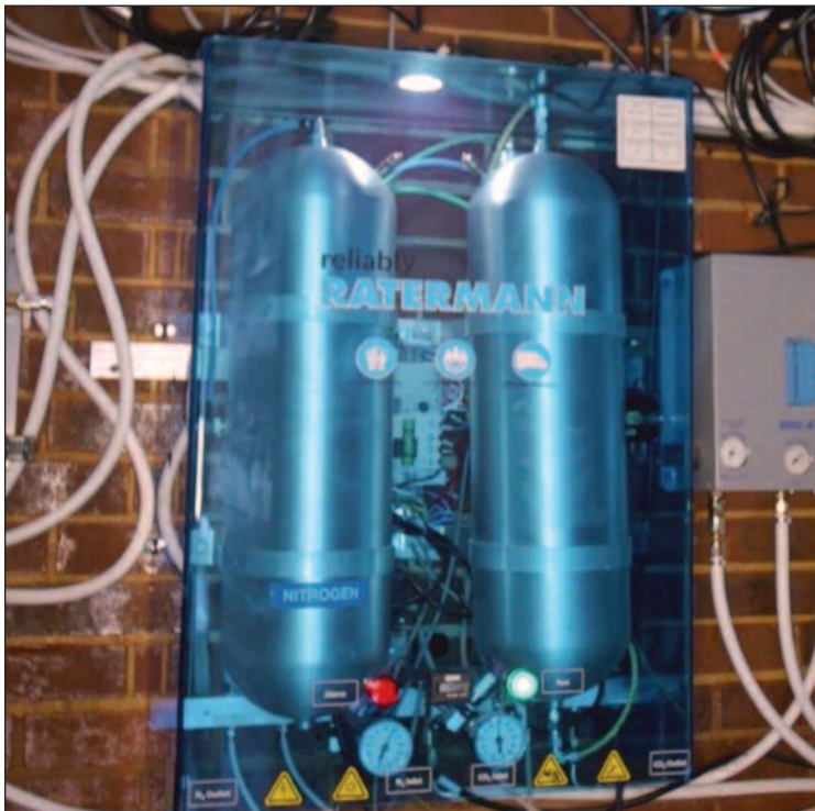
Above (Part # BRW-NG40) is the 40 Cu. Ft. Nitrogen Generator.
