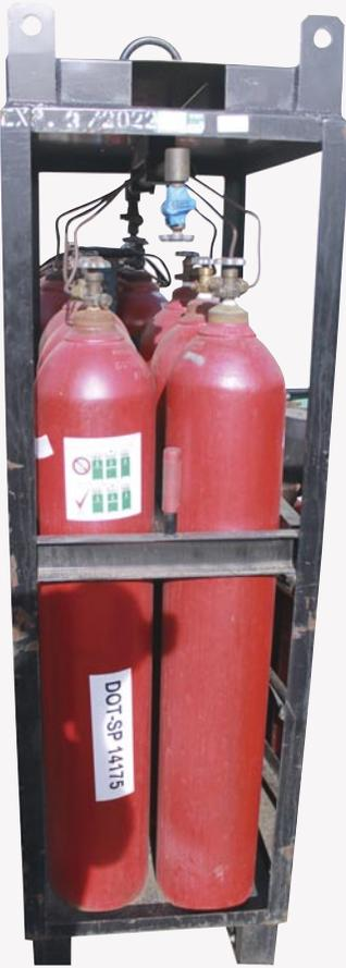
Photo example of an Used Cradle Rigid Manifold style
