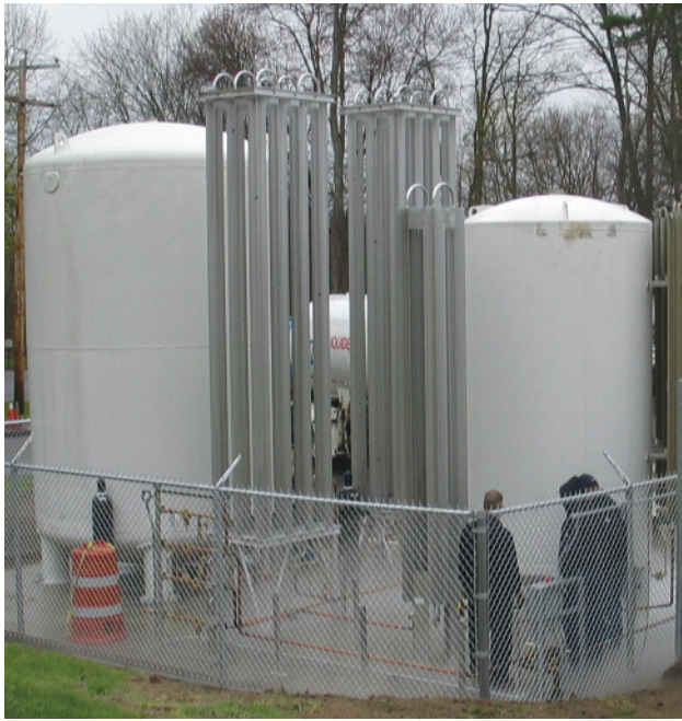
Supergap™ Ambient Vaporizers (Model TF1215-HF-SG) being installed in a hospital in North Andover, MA.
